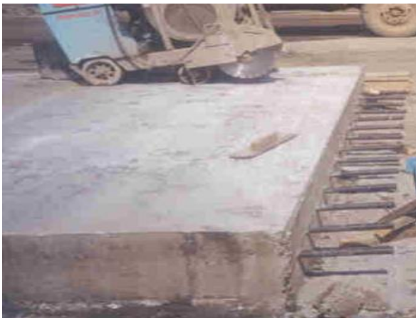
Photo 1: Dowel Bars at Transverse Joint
