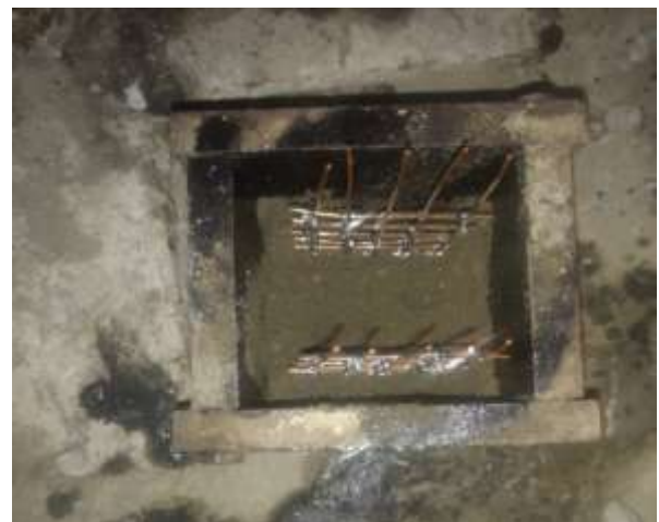
Fig 2: Copper Rods Mesh placed during casting
