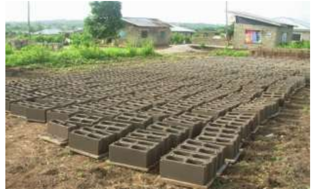
Fig 2.3: Newly moulded blocks ( Sources: http://land-for-sale-in-ogun-state.blogspot.com/2014/11/cost-of-making-blocks-vs-buying-blocks.html . Accessed 09 July 2018)
