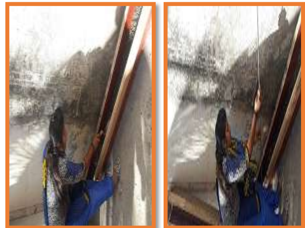
Fig 2: Pouring of Concrete 1 st Layer and Lying of Skeleton Steel
