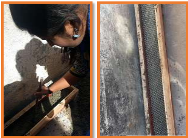
Fig 4: Pouring of Concrete and Mesh 2 nd Layer
