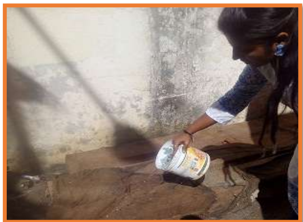
Fig 6: Curing Process for 28days
