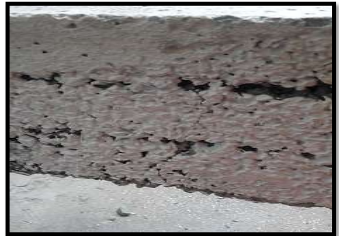
Fig -11: Flexural Test Crack
