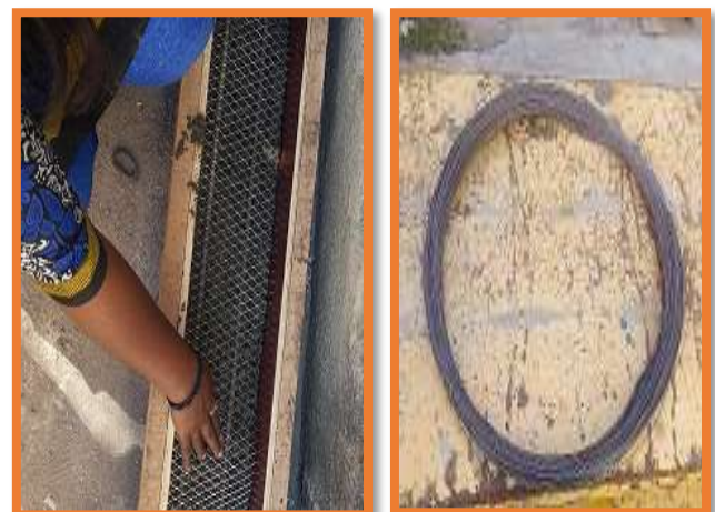
Fig 3: Pouring of Mesh 1 st Layer with Binding Wire
