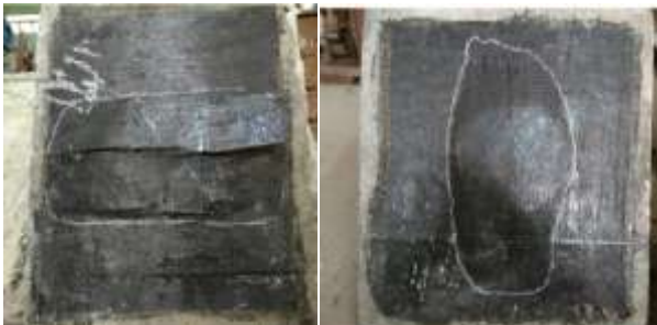
Fig 9: Failure pattern of CFRP wrapped rehabilitated slab.
