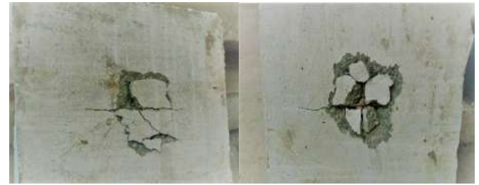
Fig. 7: Failure pattern of control slabs
