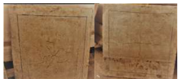
Fig 8: Appearance of First crack.
