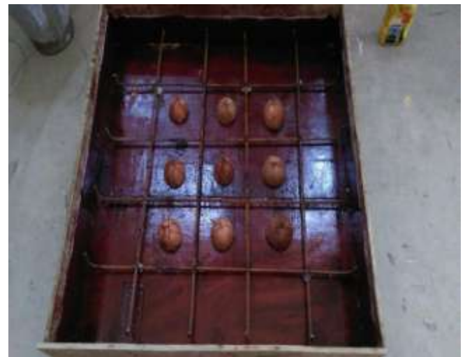
Fig 1: Coconut shell arrangement in filler slab
