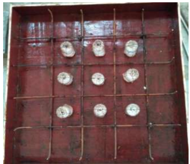
Fig 2: PET bottle arrangement in filler slab
