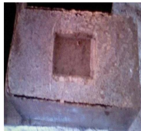
Fig 7: Failure Pattern of Blocks
