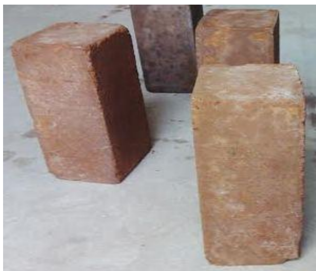
Fig 9: Efflorescence on Blocks
