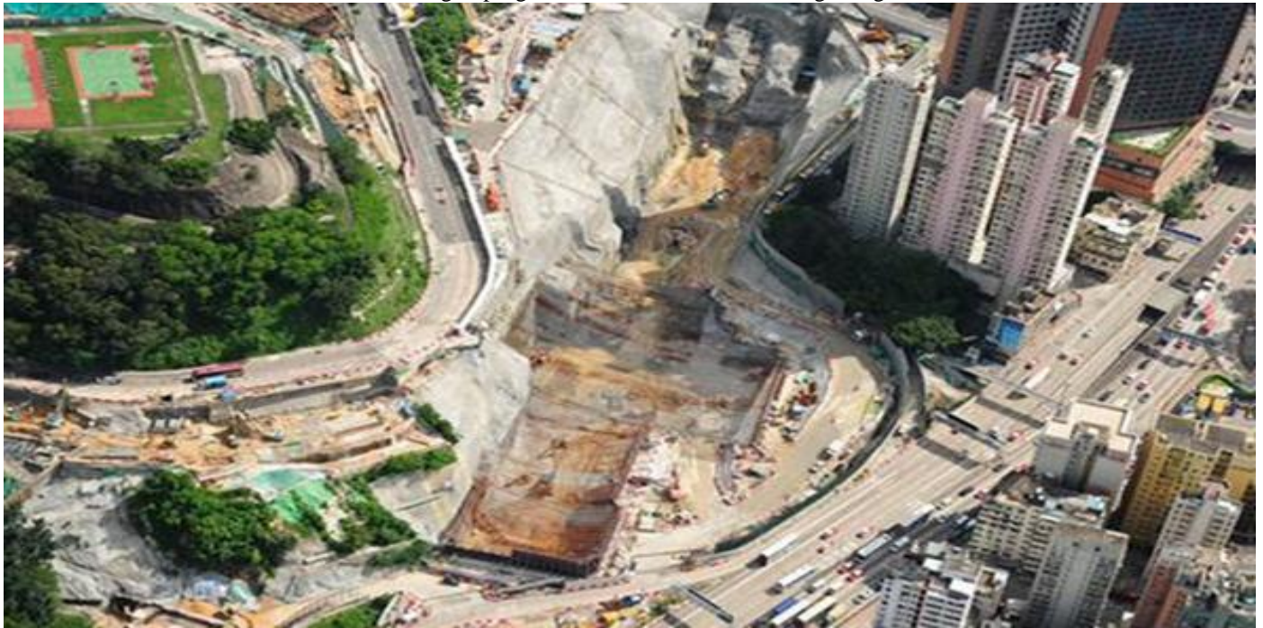
PROGRESS OF EXCAVATION IN HONG KONG
