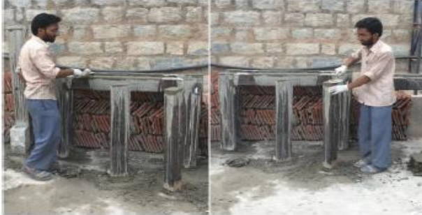
Fig 2: Finishing to the concrete exposed surfaces of frames and column.
