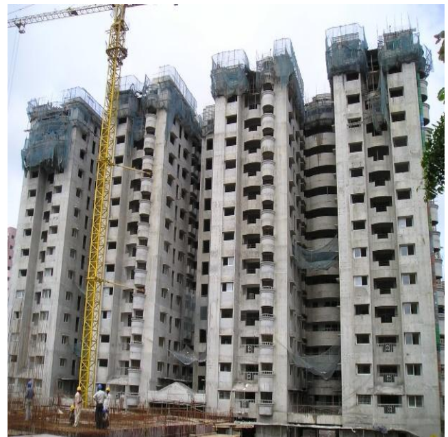
Figure – 4: Structure done with SCC with crushed sand and SNF admixture
