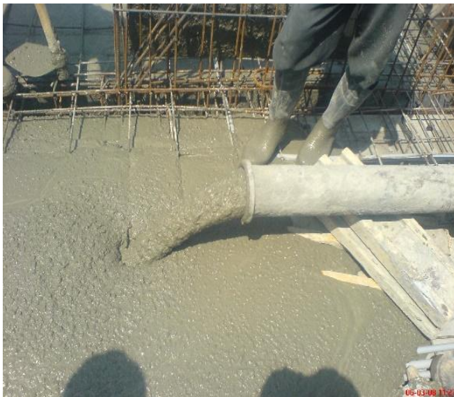
Figure – 3: Pumping of SCC
