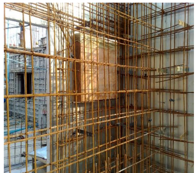
Figure – 1: Congestion of reinforcement along with electrical distribution box
