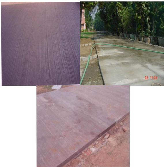
Figure 10 Broom Textured Surface (Thickness less than 40 near Director's Office))
