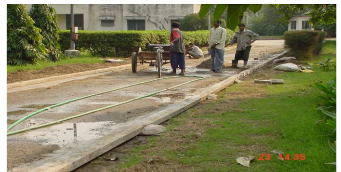
Figure 7; Form work Ready for Concreting over Existing Bitumen road, (levelling was carried out with lean concrete to adjust the crown in the middle of the road, PQC Thickness 75 mm with 1mX1m joint cutting)
