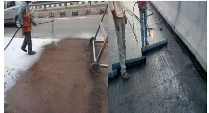
Figure 5 Insitu laying of SAMI layer
