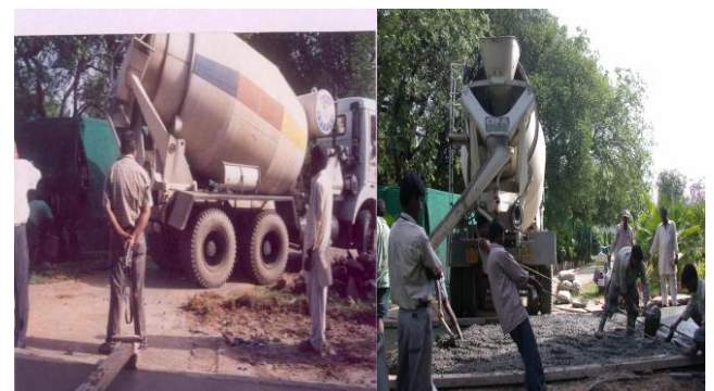
Figure 7; Form work Ready for Concreting over Existing Bitumen road, (levelling was carried out with lean concrete to adjust the crown in the middle of the road, PQC Thickness 75 mm with 1mX1m joint cutting)
