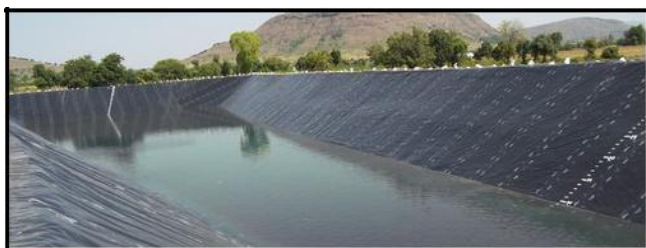
Fig -26: Water Storage during Monsoon Seasons by Geomembrane
