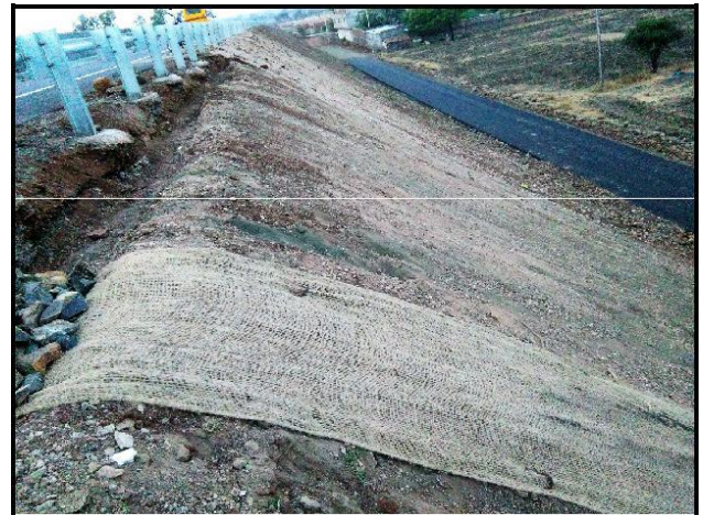
Fig -23: Placing of Natural Geotextile on Steep Slope.
