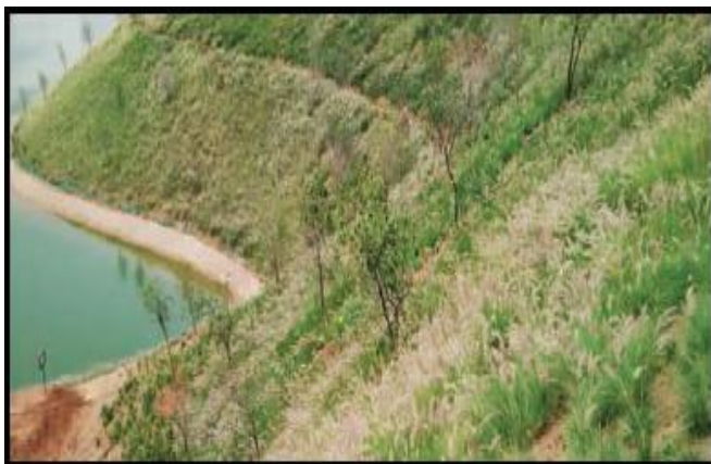
Fig -33: Development of Vegetation through Infilled StrataWeb™ on Slope
