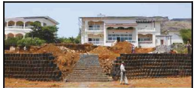
Fig -35: Gravity Retaining Wall construction using StrataWeb™.
