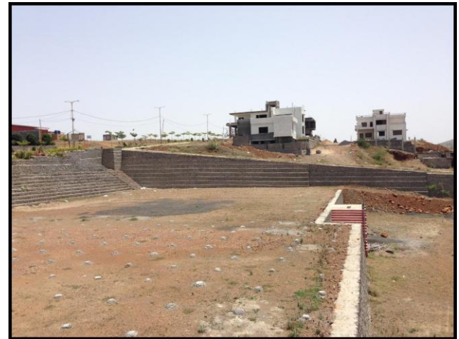
Fig -12: Developed Outdoor Sports Complex using Wrapped around Reinforced Soil Walls
