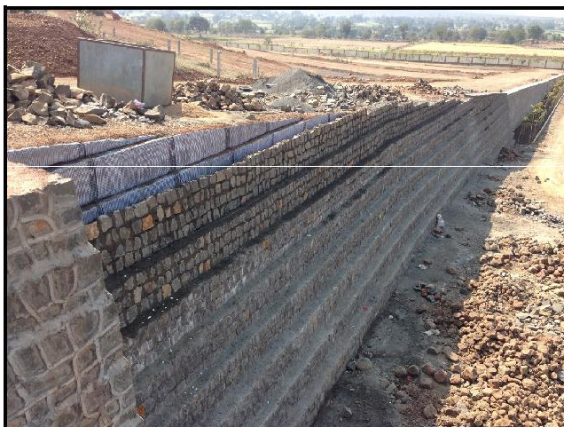
Fig -11: Construction of Wrapped around Reinforced Soil Walls using polyester geogrids
