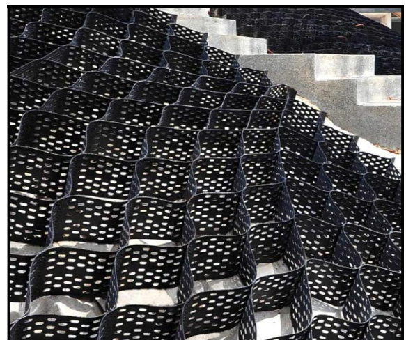
Fig -27: Perforated PE Geocells
