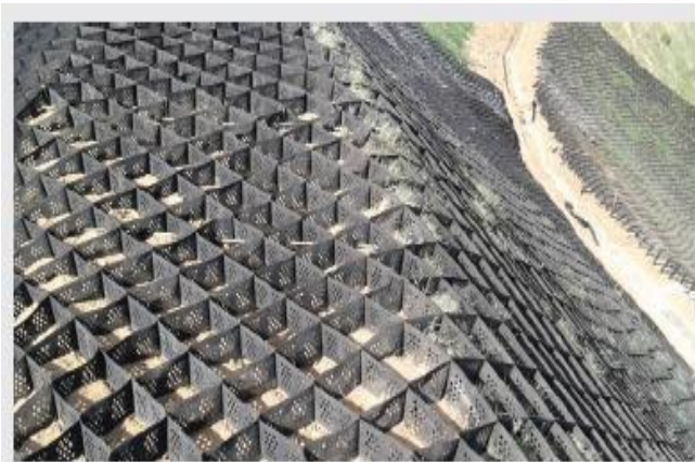
Fig -31: Placing of StrataWeb™ on Slope
