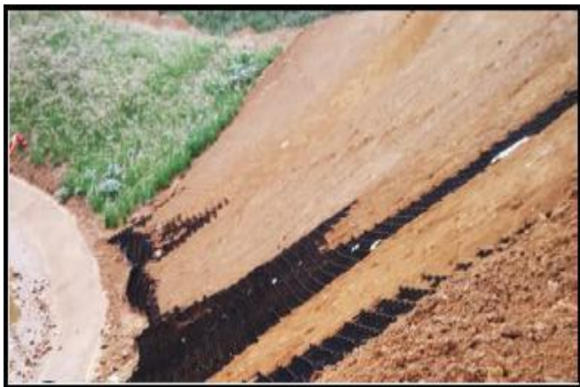
Fig -32: Infilled StrataWeb™ on Slope
