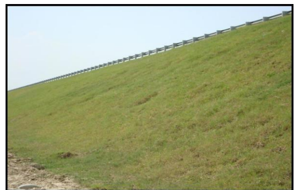
Fig -24: Development of Vegetation on Steep Slope using Natural Geotextile.
