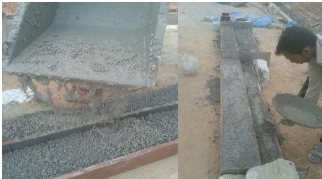
Plate 8: Casting and finishing of Light weight concrete
