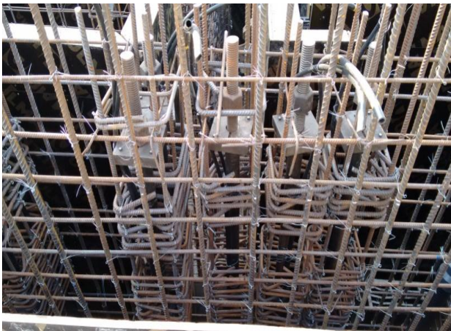
Fig 9 - Site Photo of Vertical Post Tensioning
