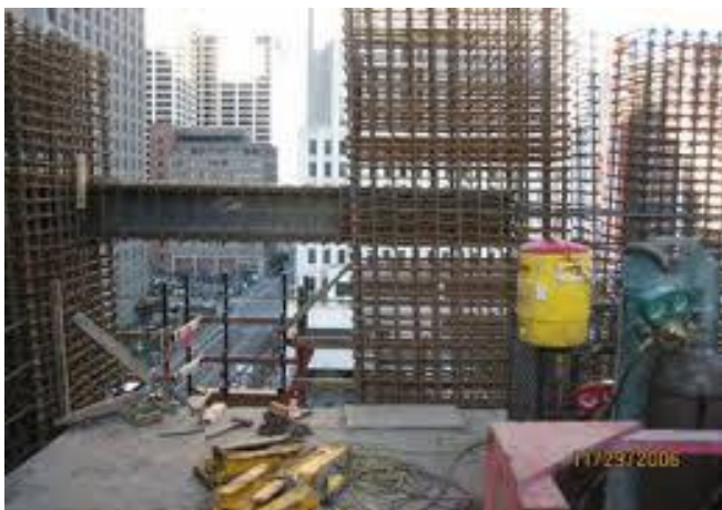
Fig 11 - Steel Coupling Beam
