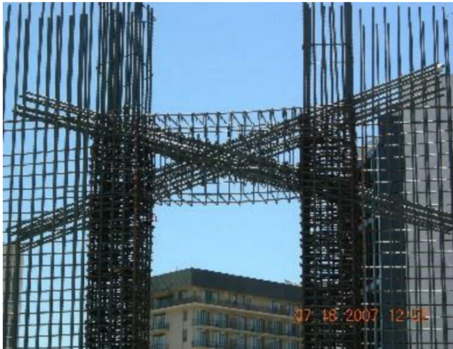
Fig 10 - Coupling Beam Reinforcement
