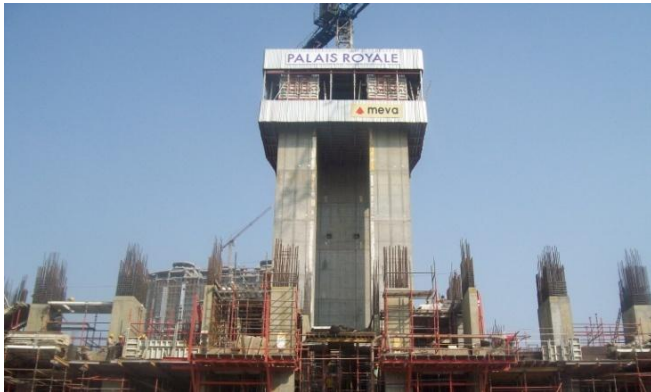
Fig 4 - Climbing Formwork
