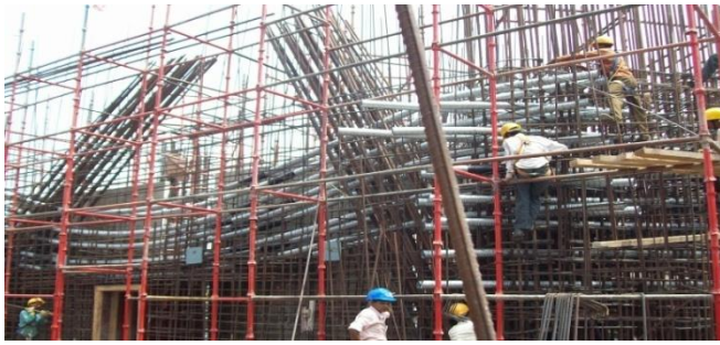
Fig 5 - Transfer Girder Embedments
