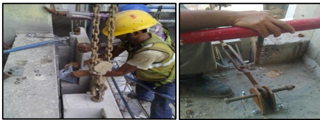
Fig -11: Bracket Fixing & Alignment
