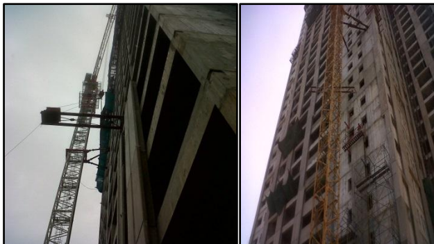
Fig -12: Tower crane Anchorage b/w precast panels
