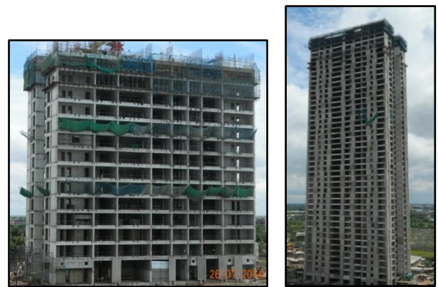
Fig- 4: Towers – Without & With Precast Panels
