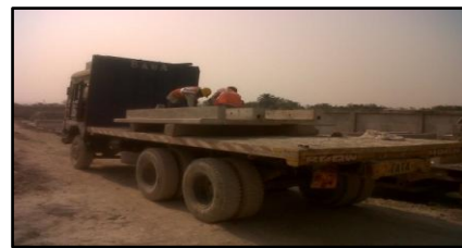
Fig -8: Transportation of precast Panels
