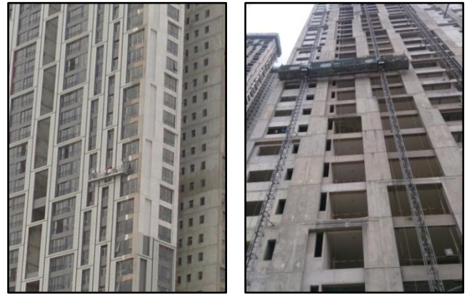
Fig -13: RSP/MCWP for Finishing Works
