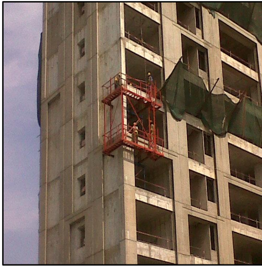
Fig -10: Working Platform for Corner Panels
