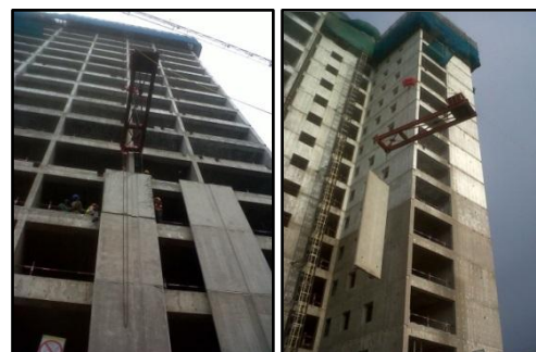
Fig -9: Erection Using Cantilever strong back
