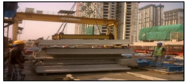
Fig -7: Typical Handling Arrangement at Yard
