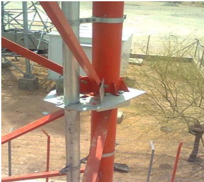
Figure 1: Split flange stiffened coupling plate
