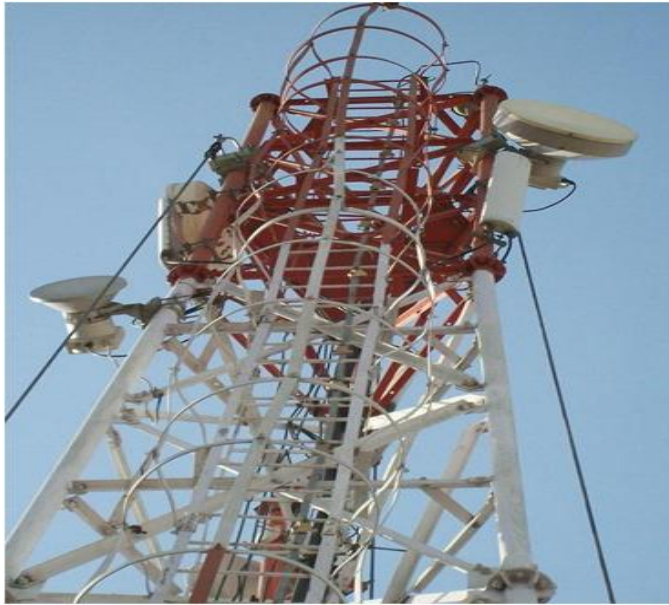
Figure 4: RTT strengthening using guy ropes
