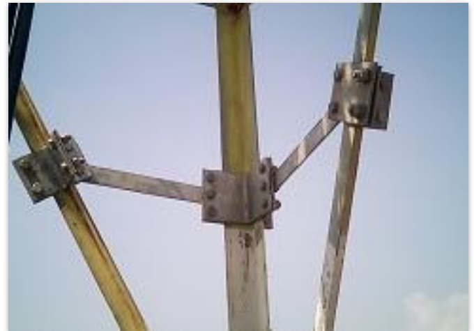
Figure 3: Main Leg Strengthening
