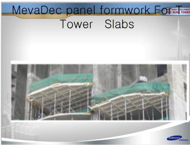
Fig-14: Tower Slab Formwork and FRP shuttering
