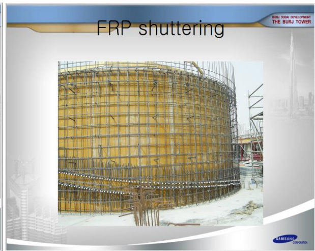
Fig-14: Tower Slab Formwork and FRP shuttering
