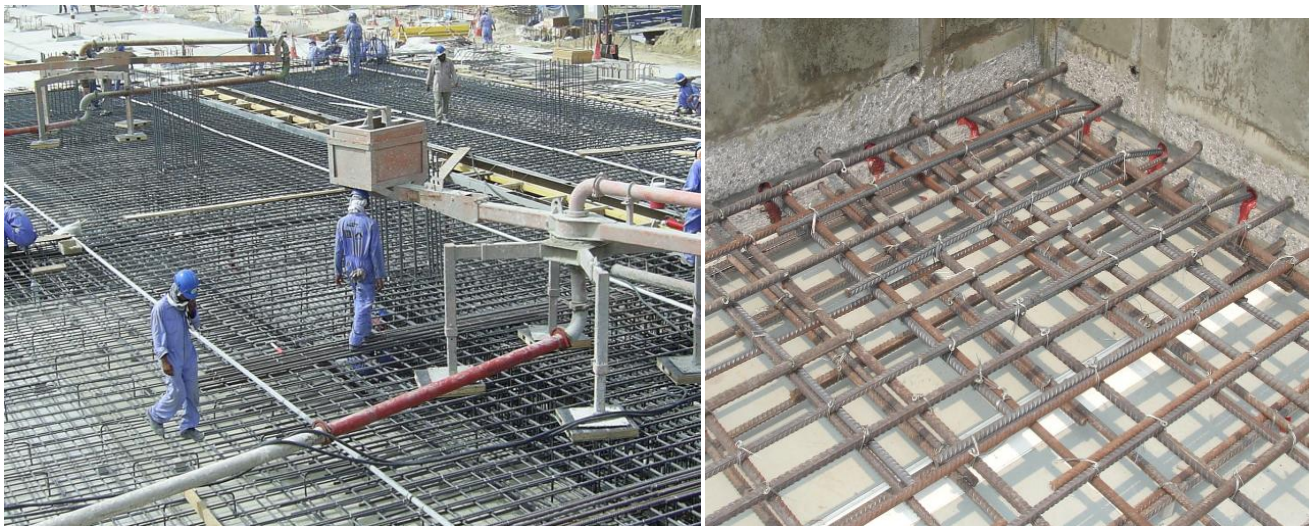
Fig- 22: Rebar: Mat Foundation and Tower Slab
