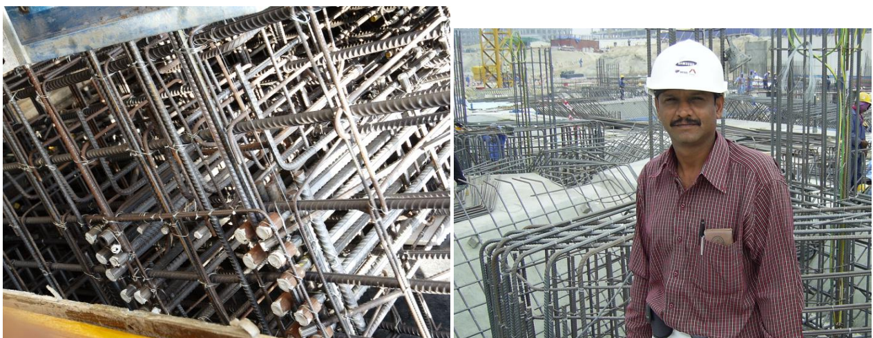
Fig- 23: QC Inspection: Mat Foundation and Tower Beam
