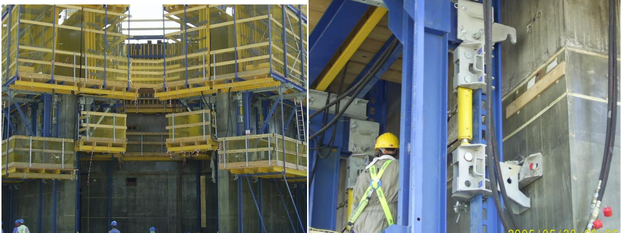
Fig- 21: Auto Climbing Formwork
