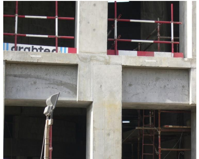
Figure 12. Walking column detail of Cayan Tower.
