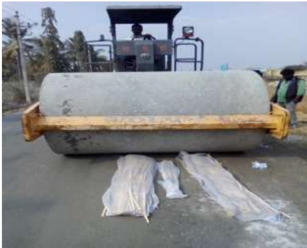
Fig 4 Crushing of bamboo strips by roller
