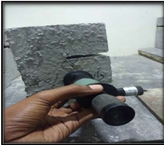
Fig 5: Crack Width by Filar Microscope
