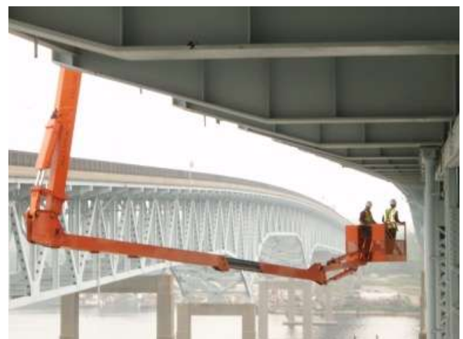
Fig 1- Site of manual bridge testing
