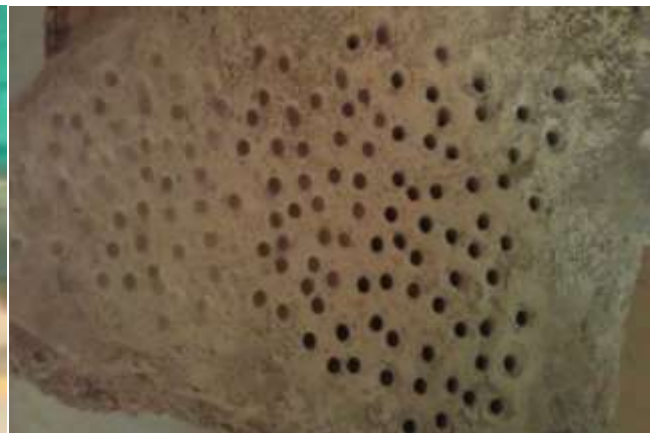
Fig - 2: Holes left in the concrete debris after sample collection
