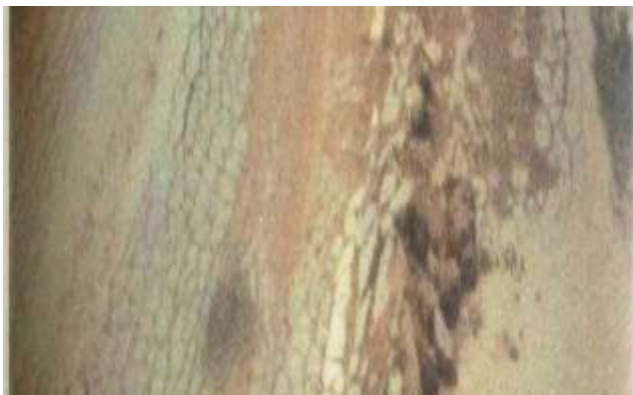
Figure 1: Longitudinal Cracks On A Highway Pavement At Oniyale, Ifo Locality.
