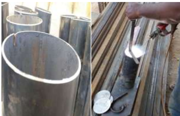
Fig-1: Machine cut steel tube and welding of stiffeners
