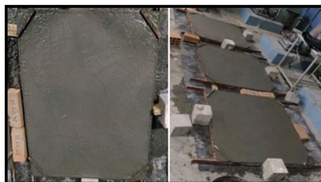
Fig -1: Casting of GPC & M-20 concrete OPC Slabs
