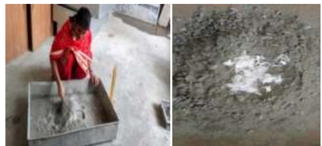
Fig 3: preparing concrete mix and adding fiber to concrete
