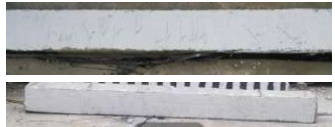
Fig 12. Crack pattern and debonding occurred in SB-1 beam
