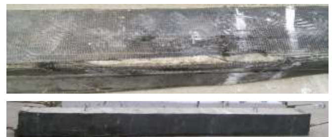
Fig 14. Crack pattern and full debonding occurred in SB-3 beam.
