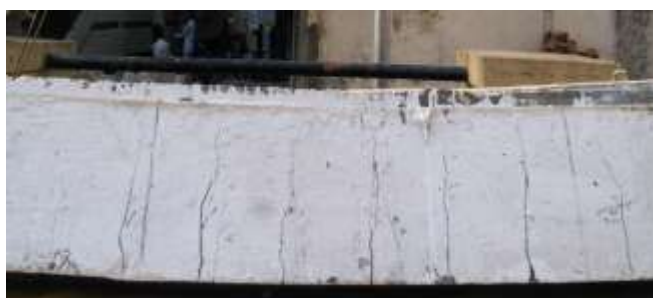
Fig 11. Crack pattern in control beam
