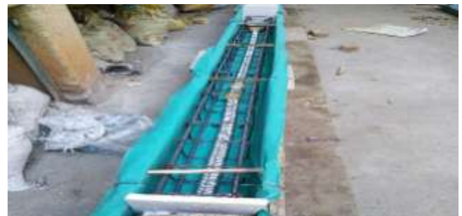
Fig 2 Reinforcement and its cage
