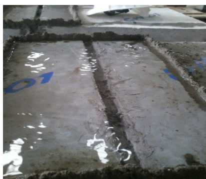
Fig-9: Trial 5 joint
