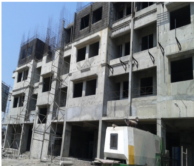
Fig 2 : Construction using ALUFORM system.
