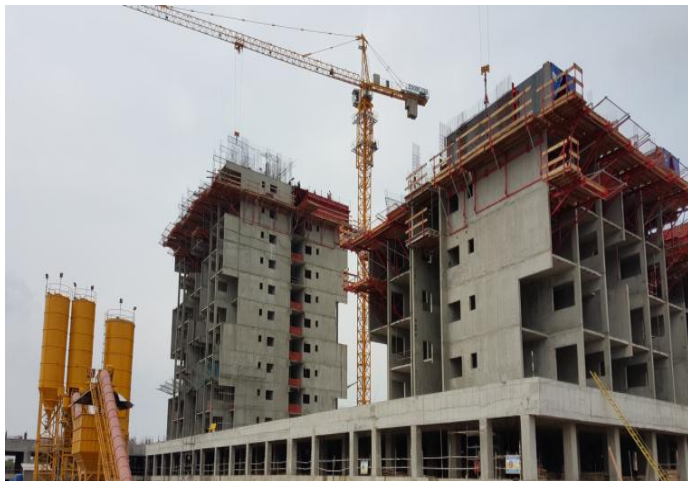
Fig 5: Construction using TUNNEL formwork
