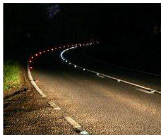
Figure 5. Shows how the road looks like after reflectors being installed
