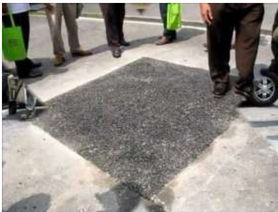
Figure 6. Shows how it looks like after repairing the pothole
