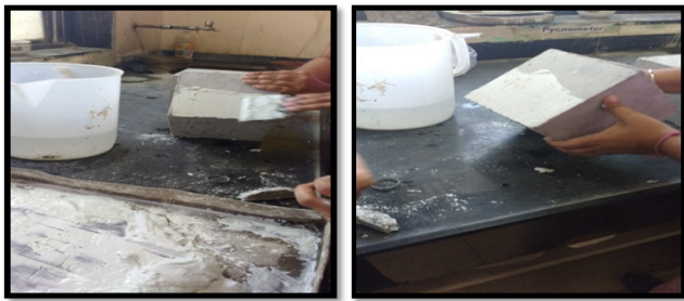
Coating of cubes by Dr. Fixit (bio concrete cubes)
