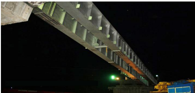
Fig -1: I section girder on ROB.
