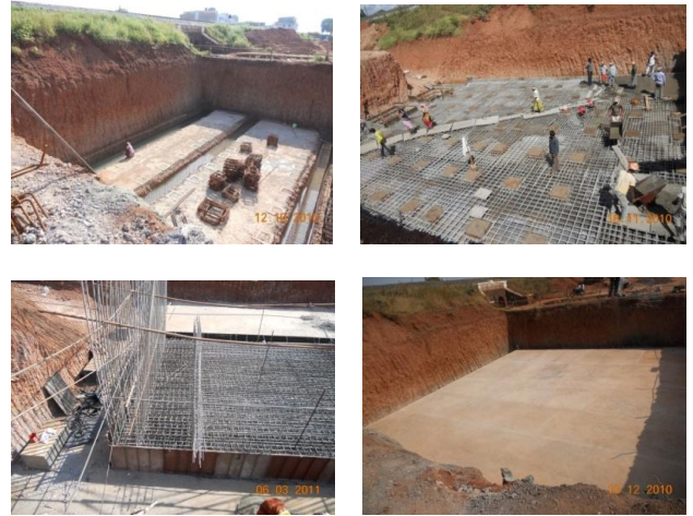
Fig -3: Foundation of road in Box Pushing in RUB.
