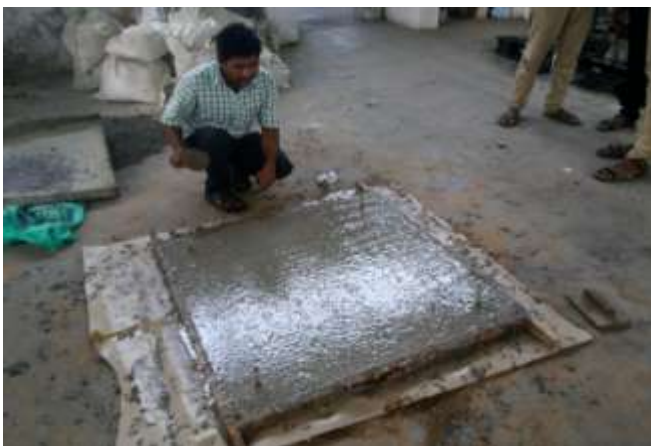
Fig .10: Shows the Casting of GPC Slab
