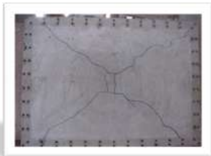
Fig 19 : Actual Crack on bottom surface for a Fixed Slab (Panel – 1) ( F_1 ) Subjected to UDL
