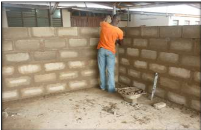
Fig - 1 (a): Sandcrete block wall
