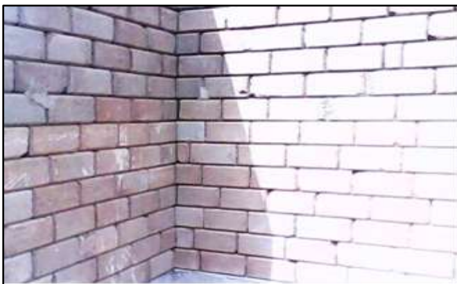
Fig - 1(b): Interlocking block wall
