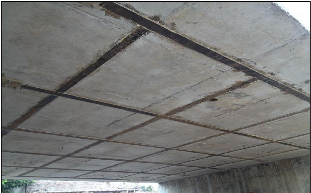
Fig. 8 Strengthening with Non Prestressed FRP laminates at bottom of slab of ROB at Markapur (Courtesy:- M/s R & M International Pvt Ltd)
