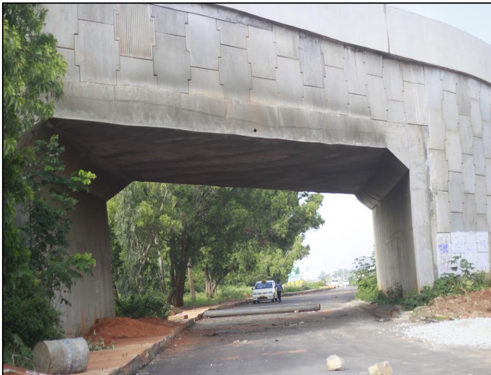
Fig. 6 Post strengthening of skew Slab Bridge (Courtesy:- M/s R & M International Pvt Ltd)
