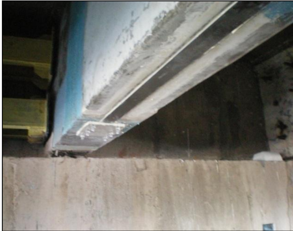
Fig. 3 CFRP prestressed laminates in girders [9] (Courtesy:- M/s R & M International Pvt Ltd)
