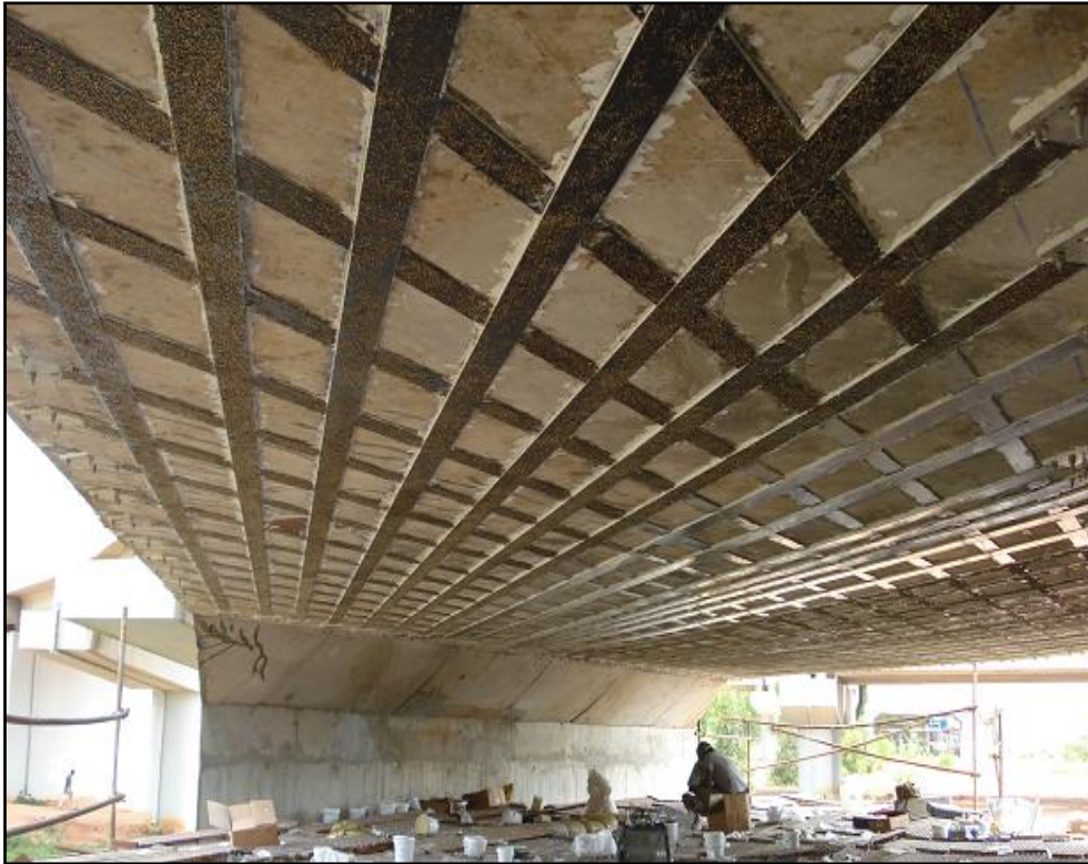
Fig. 5 Prestressed FRP laminates at bottom of skew slab bridge (Courtesy:- M/s R & M International Pvt Ltd)
