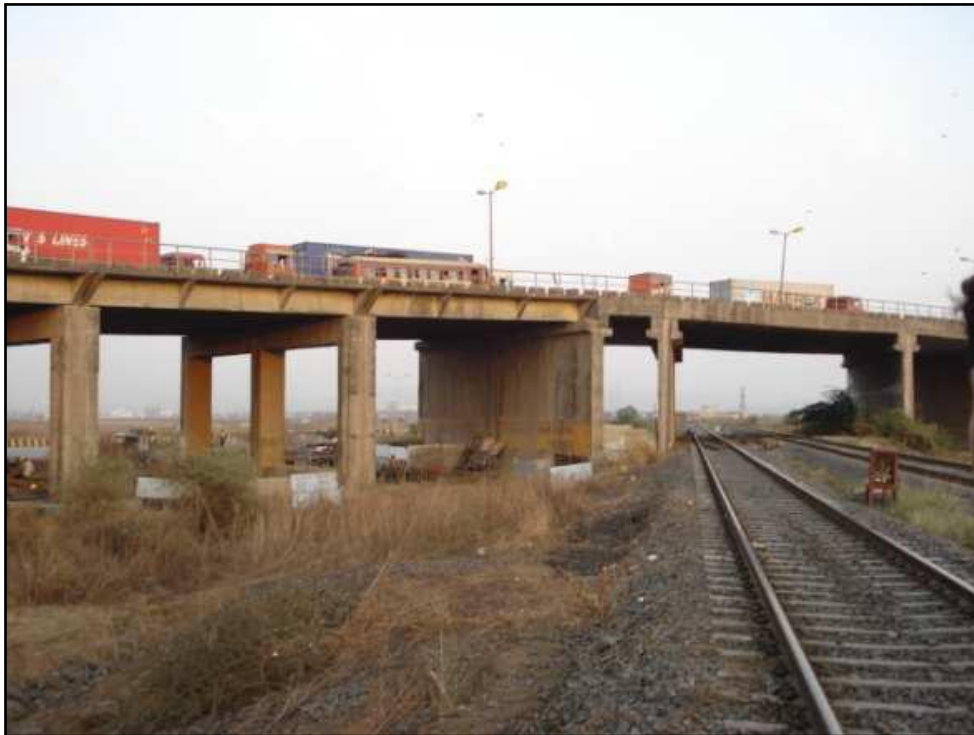
Fig. 1 Rail Over Bridge (ROB) at JNPT [9] (Courtesy:- M/s R & M International Pvt Ltd)
