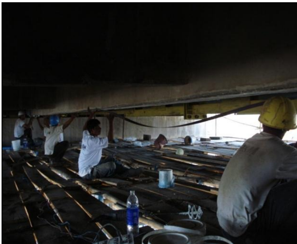
Fig.2 Bottom of girder with Prestressing of CFRP laminates in process [9] (Courtesy:- M/s R & M International Pvt Ltd)
