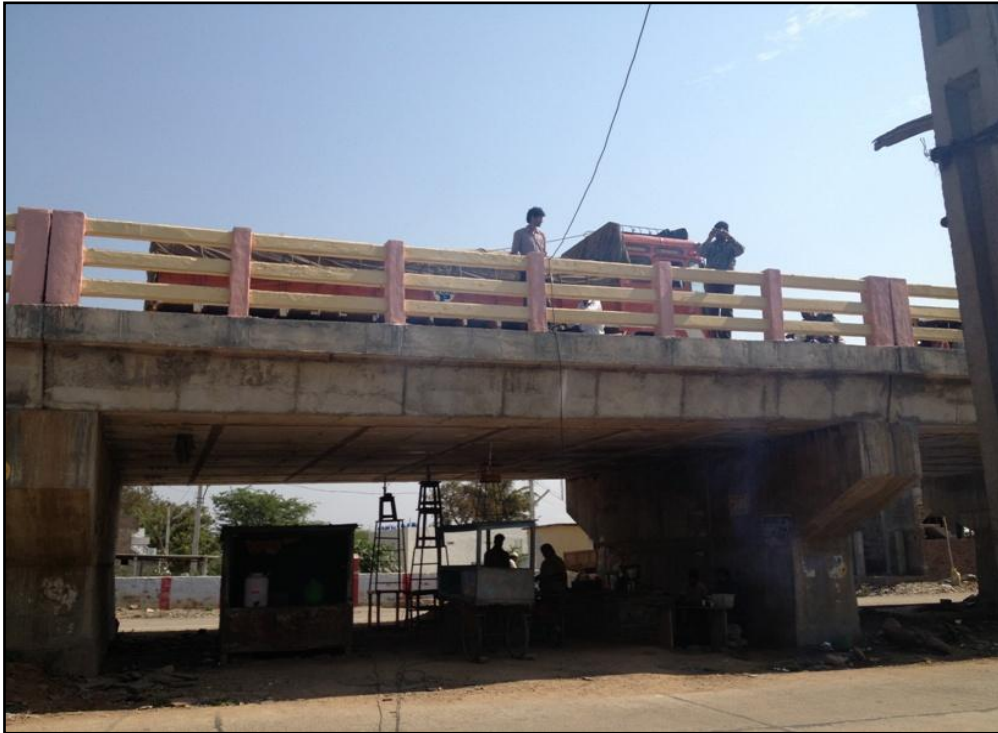
Fig. 9 Load test being carried out post strengthening of ROB at Markapur (Courtesy:- M/s R & M International Pvt Ltd)
