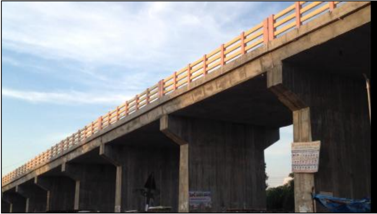
Fig. 7 ROB at Markapur requiring strengthening (Courtesy:- M/s R & M International Pvt Ltd)
