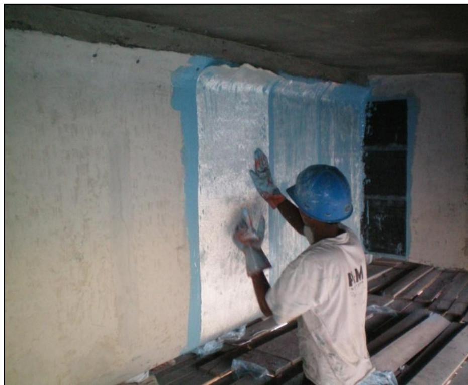
Fig. 4 FRP application on girder for shear strength increase (Courtesy:- M/s R & M International Pvt Ltd)
