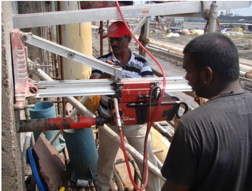
Fig. 3 Core extraction in progress
