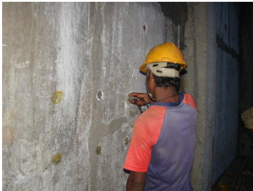
Fig. 2 UPV Test in Progress
