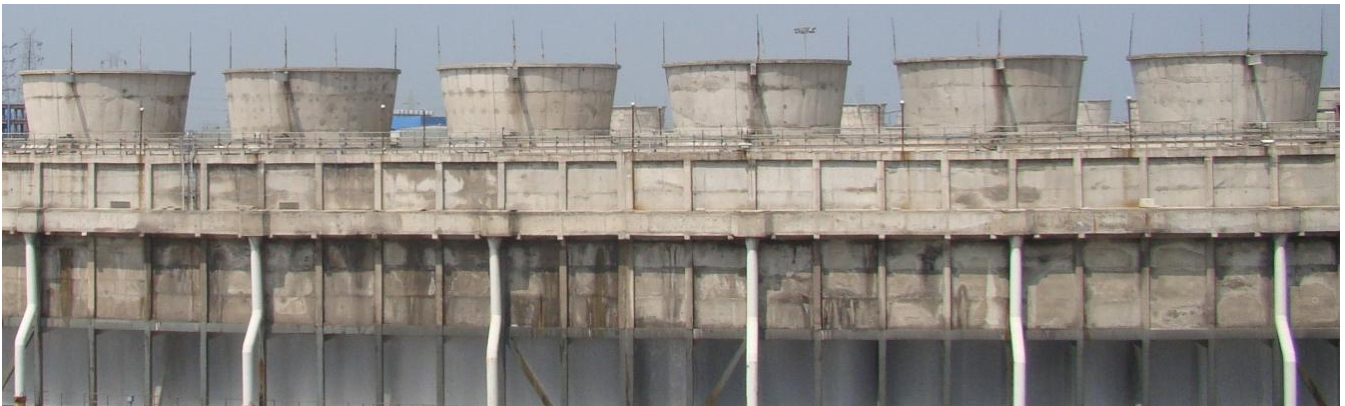
Fig.1 Typical view of IDCT
