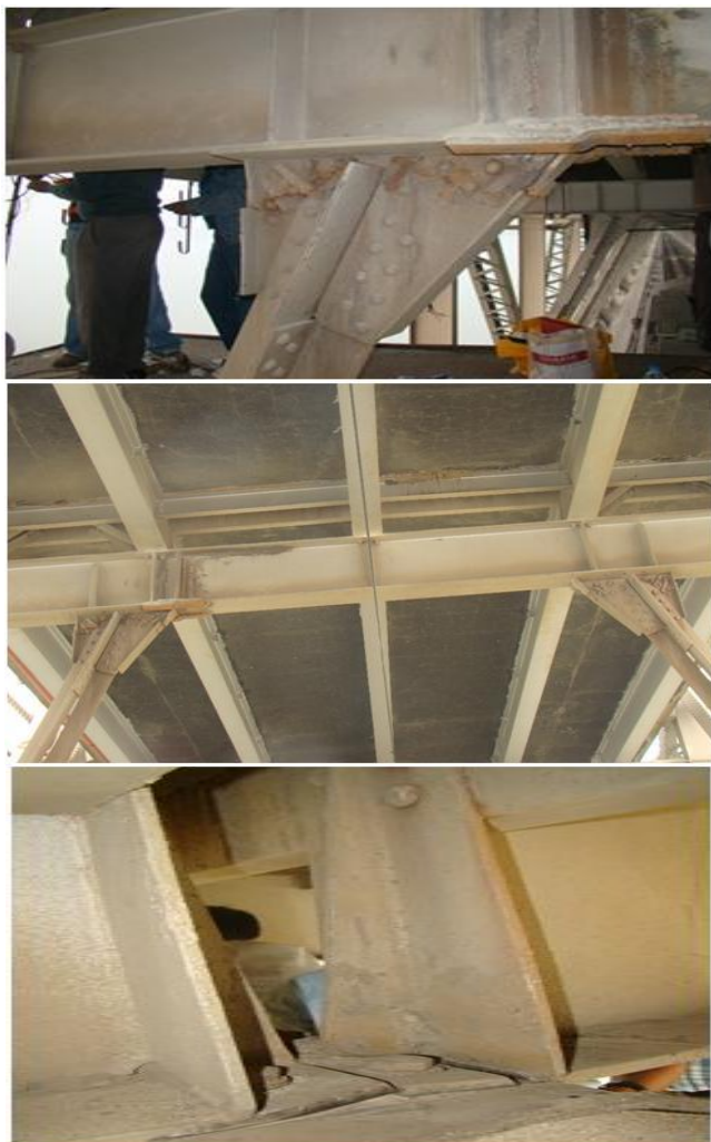
Fig.2 Damages observed in the structural members of the bridge
