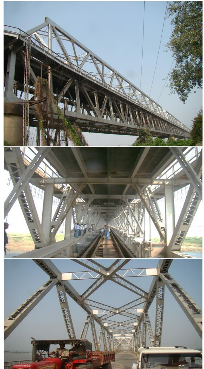
Fig.1 General view of the Open Web Girder Road cum Rail Bridge
