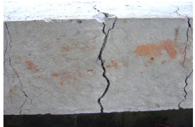
Fig. 4. Failure mode of reference beam
