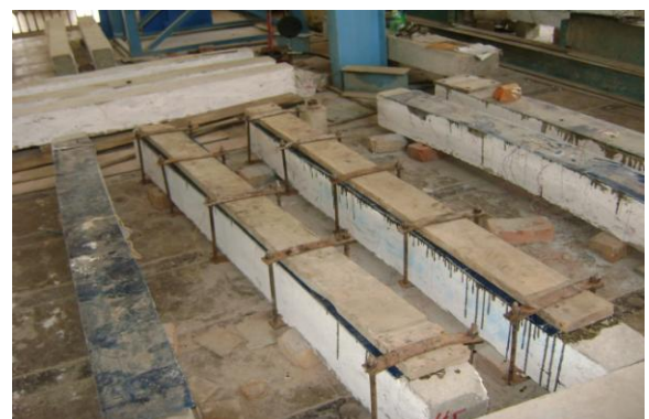
Fig. 3. GFRP laminates pasted at tension side of RC beams
