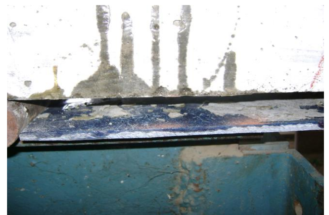
Fig. 5. Failure mode of beam strengthened with symmetric cross-ply laminate
