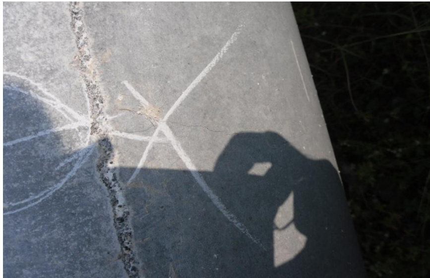
Figure 3: Surface Cracks for Pole with Glass Fibers
