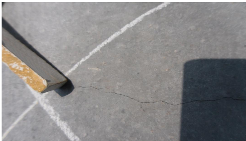
Figure 2: Surface Cracks for Pole without Glass Fibers
