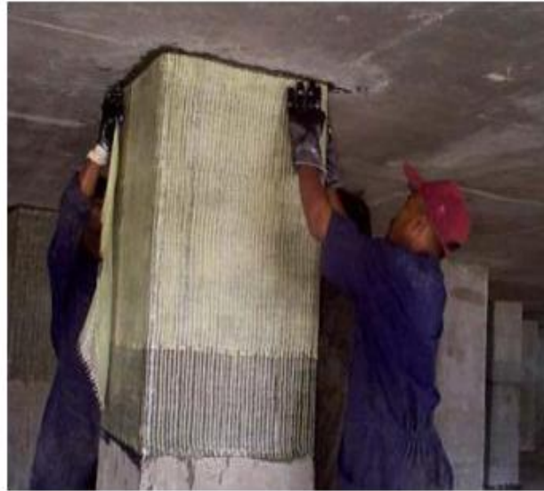
fig.6- retrofit of columns for a cryogenic tank in Gujarat, India 11 .
