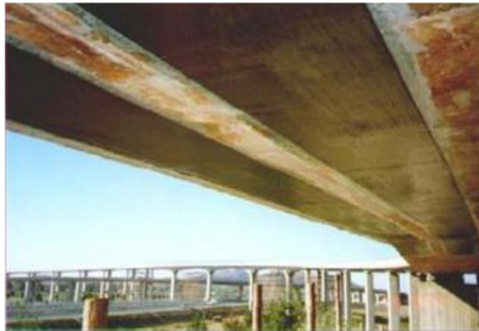
fig.4. strengthening of a highway RC bridge slab in China 11 .
