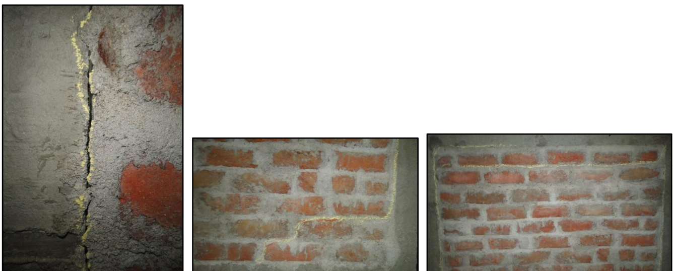
(A) Separation of mortar bond at column face (B) Stepped type of failure (C) Failure of horizontal mortar joint.
