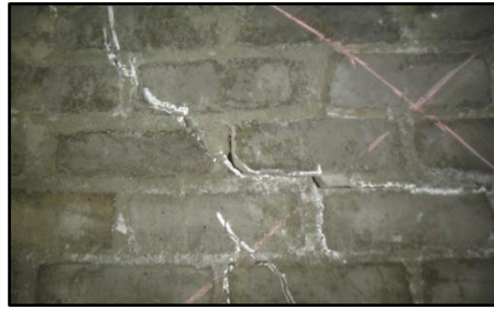
(B) Stepped Failure
