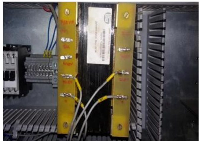
FIG-3 750VA/220VA TRANSFORMER
