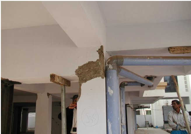
Fig 2: Failure of Column, Bhuj, during Bhuj Earthquake, 2001 [4]
