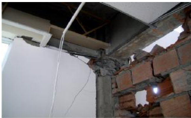
Fig 3: First Storey Corner Column Showing Damage at the Top End, Mianzhu City, during Wenchuan Earthquake, 2008 [2]
