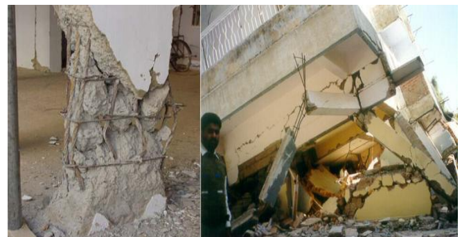
Fig 1: Failure of Column and Collapse of Structure at Bhuj, during Bhuj Earthquake, 2001 [4]
