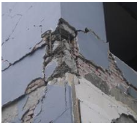
Fig 4: Damaged RC Column at the Second Storey, Dujiangyan City, during Wenchuan Earthquake, 2008 [2]
