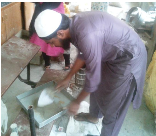
Fig 3.7: mixing of sand and cement with corresponding ratios
