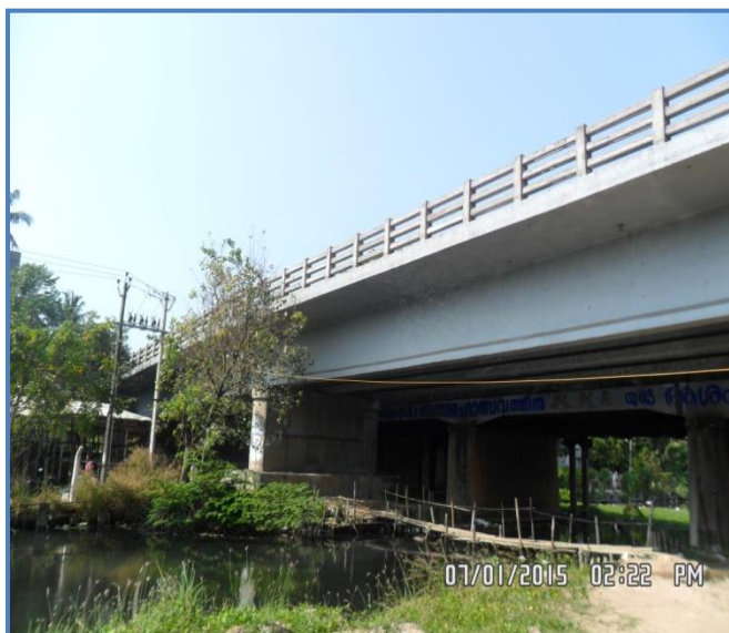
Fig -4: Bridge at Kollam
