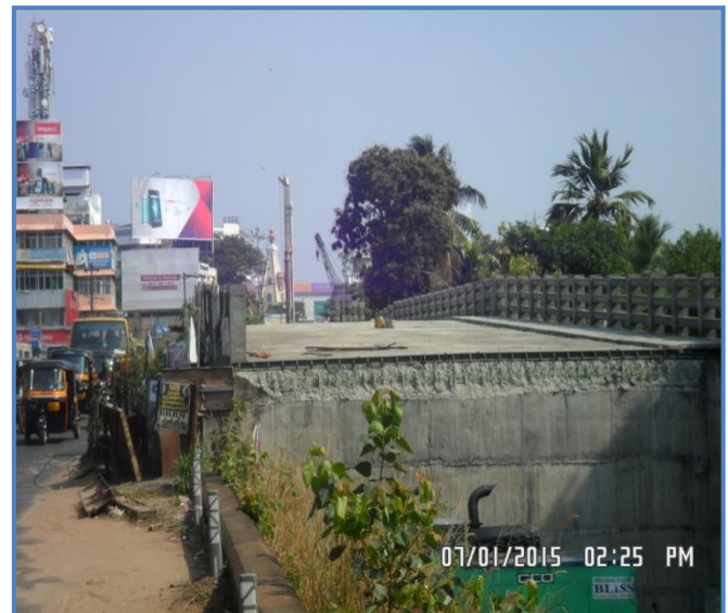
Fig -5: Kollam Bridge top view
