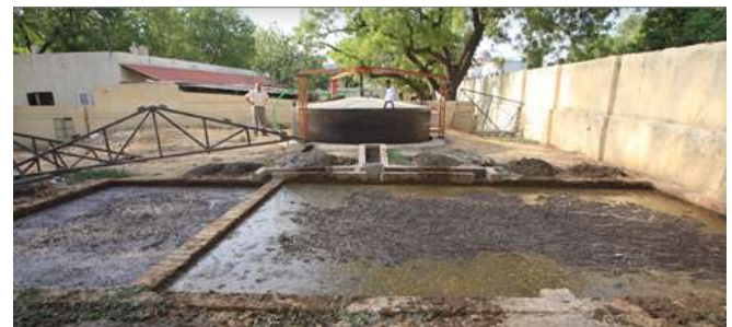
Fig -8: Storage of Biogas Power Plant
