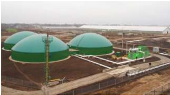
Fig -9: Site of Biogas Power Plant
