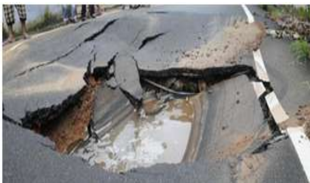
Figure 4: Damage of road due to pipeline burst.
