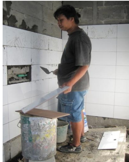
Figure 7. The ceramics dan mortar are placed on the pedestal
