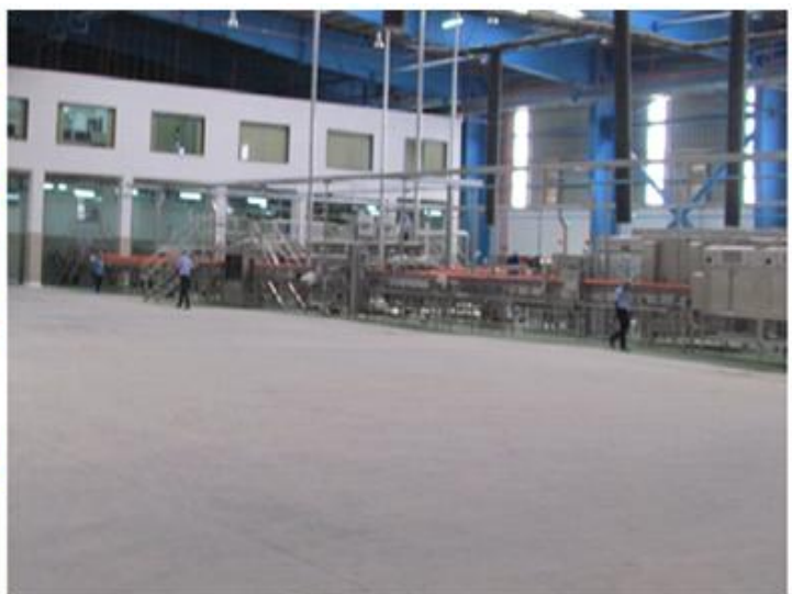
Fig 4 Steel fibre reinforced concrete slab at site after construction
