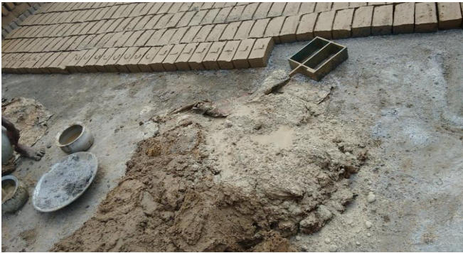
Figure -3: Fly ash stabilization
